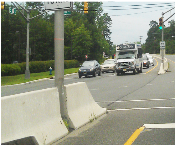
NJ State Route 37 is currently a very auto-oriented corridor with strip development lining its frontages.
