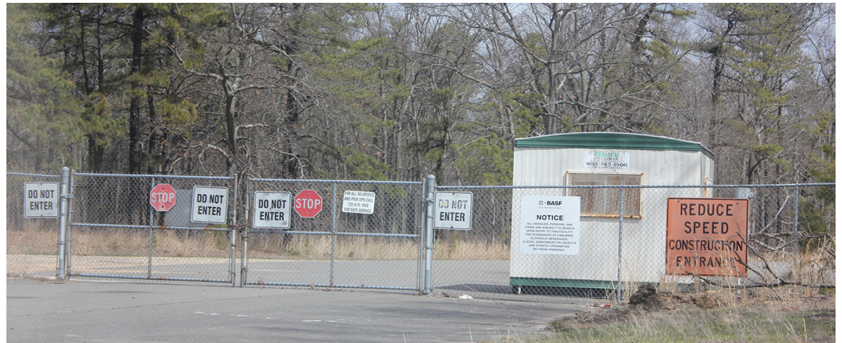
Entrance to Ciba-Geigy site, currently closed for on-going environmental remediation work.
