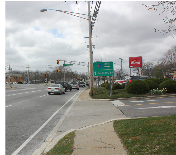
There is little pedestrian and bicycle access and connectivity along Rt. 37. Where sidewalks exist, they are continuously broken by large drive entrances
