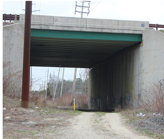
Rail right-of-way runs underneath the Garden State Parkway linking the corridor to Downtown
