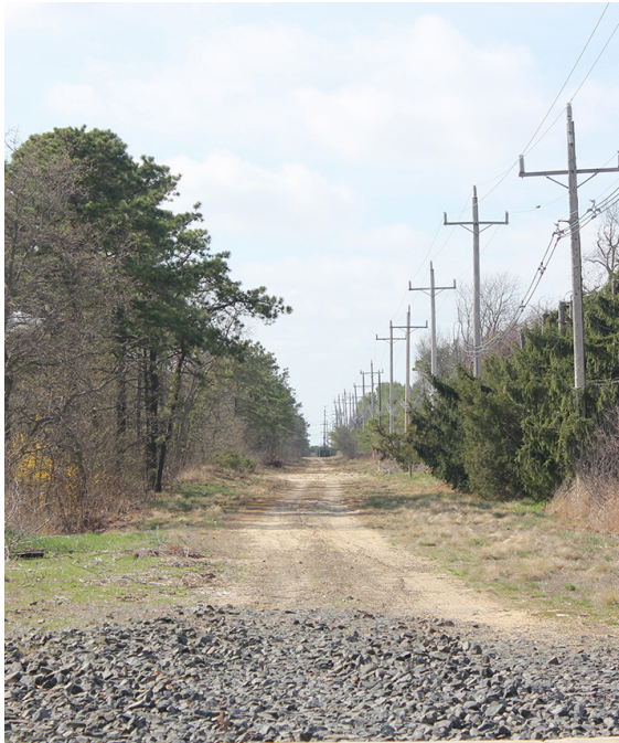
Existing Rail ROW Parallel to Route 37
